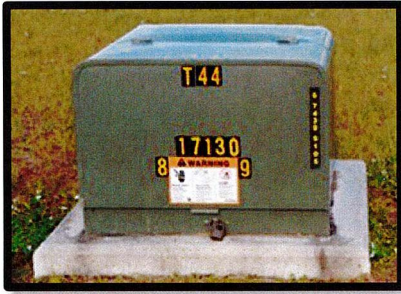
Typical Residential Pad-Mount Transformer Typical Size: 40"L x 36"W
