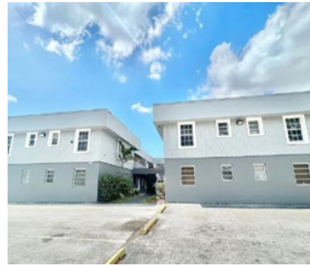
15 2846 Fillmore Street, Hollywood, FL 33020
