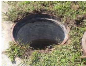
Manhole Interior Following Sand-blasting
