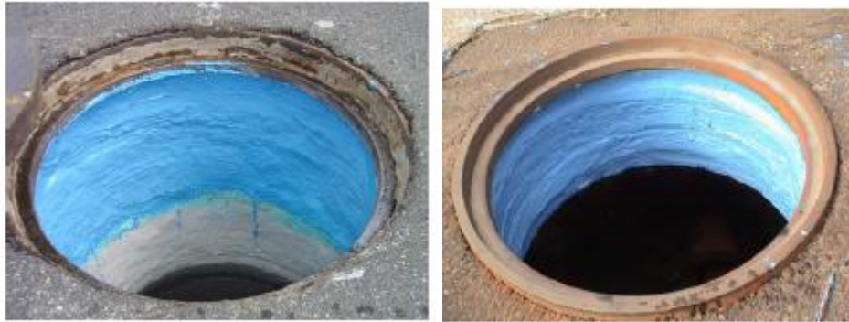
Figure 4.1 chimney seal installed.
