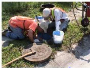
Frame & Chimney – Elastaseal® Coat
