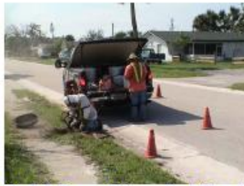
Manhole Frame / Chimney Sand-Blasted
