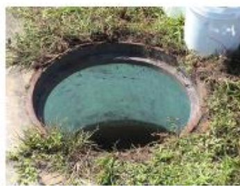
Frame & Chimney – Prime Coat
