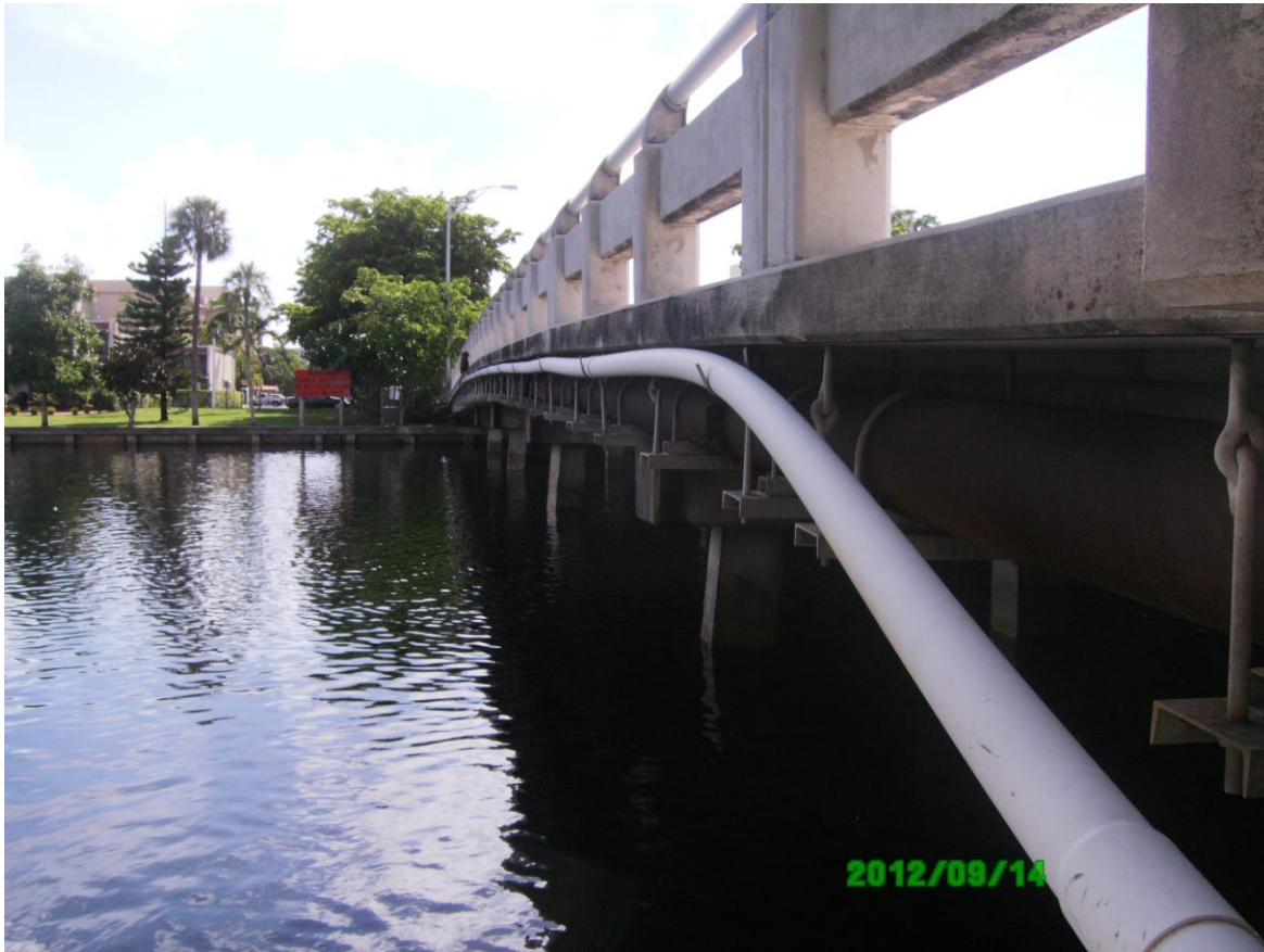
Figure 5: Existing water main and gas line attached to north side of bridge structure, facing east
