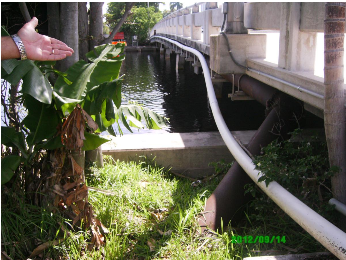
Figure 4: Existing water main and gas line attached to north side of bridge structure, facing east
