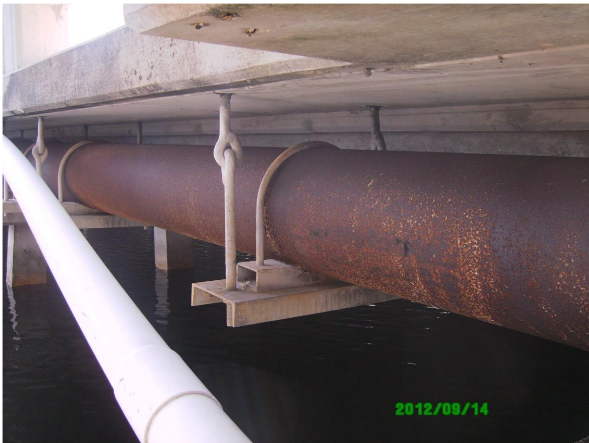
Figure 6: Close-up of water main pipe hanger
