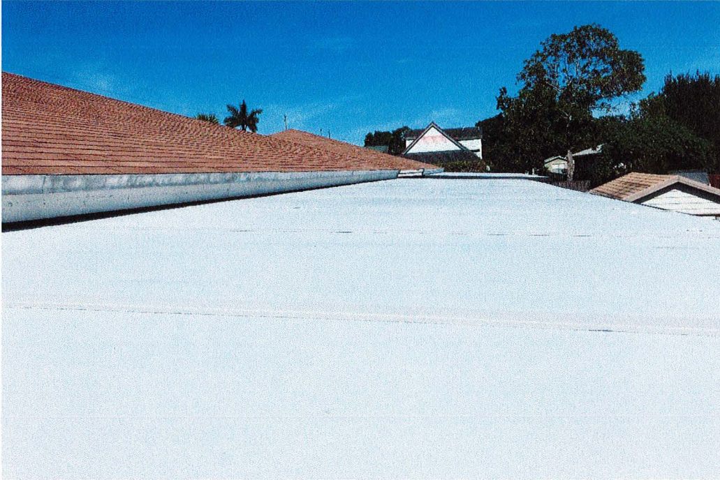
Photograph 3. Panels top view. 4 ft wide panels
