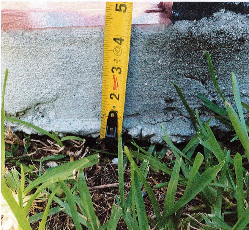
Photograph 10. 4" thick slab on grade
