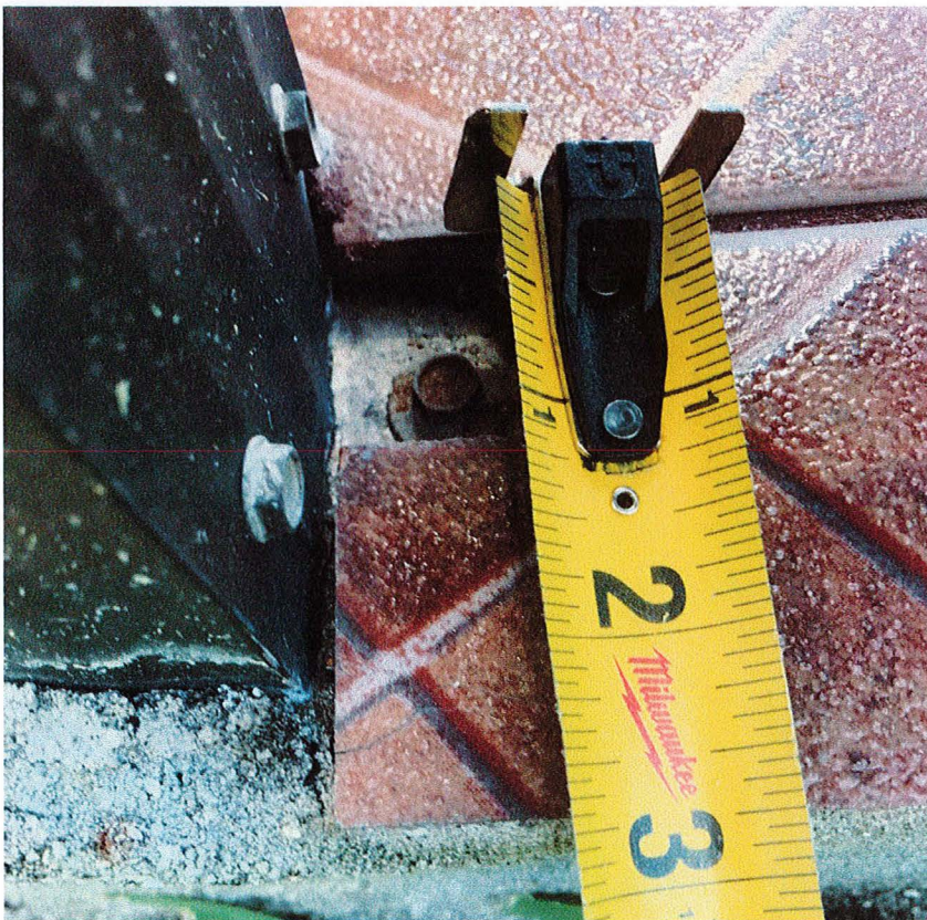
Photograph 6. Bolted connection to concrete slab
