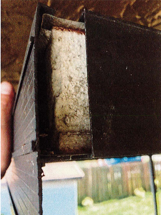
Photograph 5. Panels Cross section, 3" thick. Aluminum top and bottom sheets and insulation can be observed
