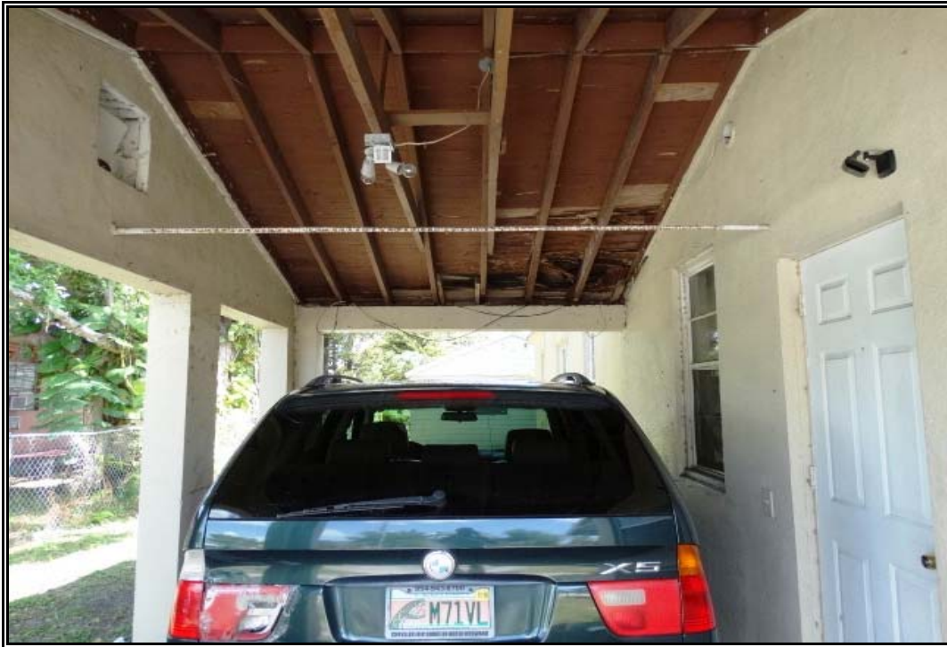
View of carport and roof damage
