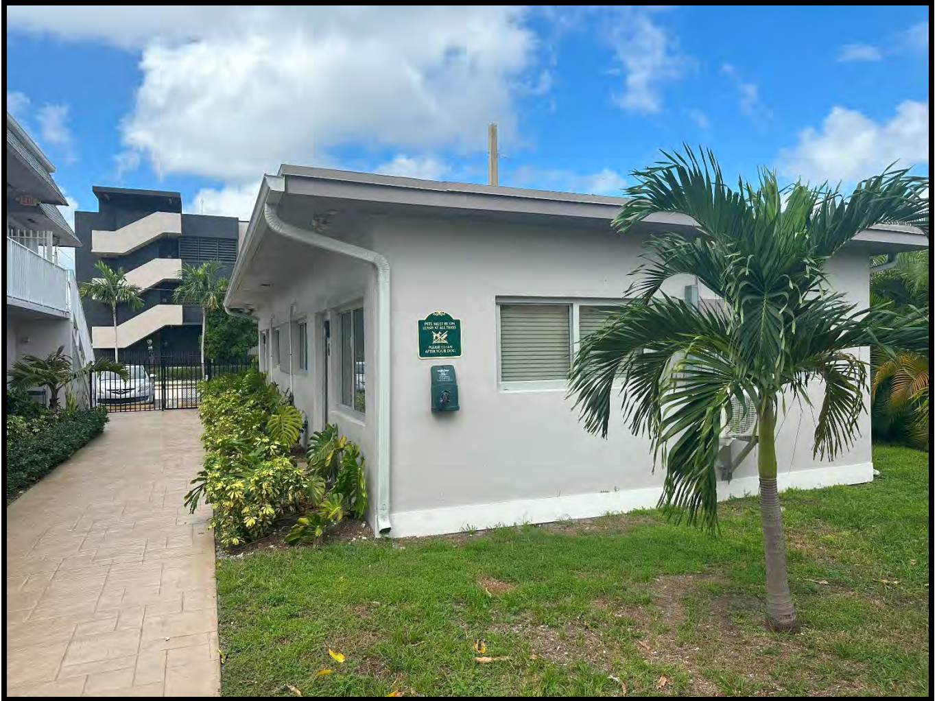
View of rear of northwest building at 415 S.E. 3rd Avenue facing westerly from courtyard
