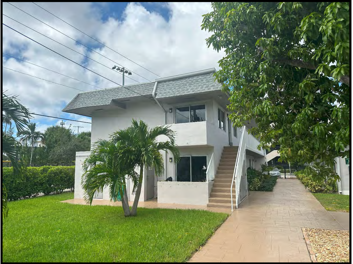
View of rear of southwest building at 417 S.E. 3rd Avenue facing westerly from courtyard
