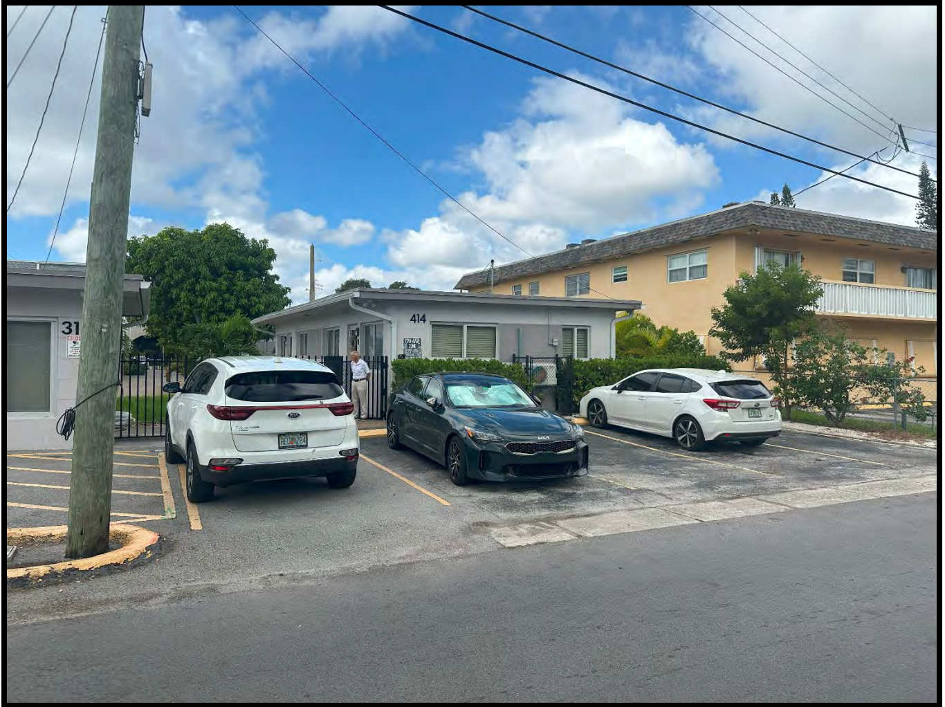
View of northeast building at 414 S.E. 4 th Avenue facing westerly from S.E. 4th Avenue
