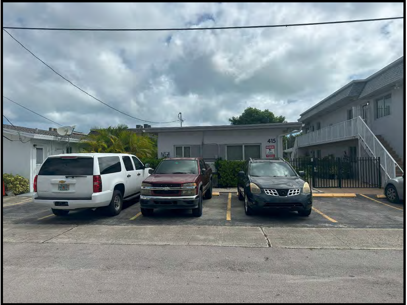
View of northwest building at 415 S.E. 3 rd Avenue facing easterly from S.E. 3 rd Avenue
