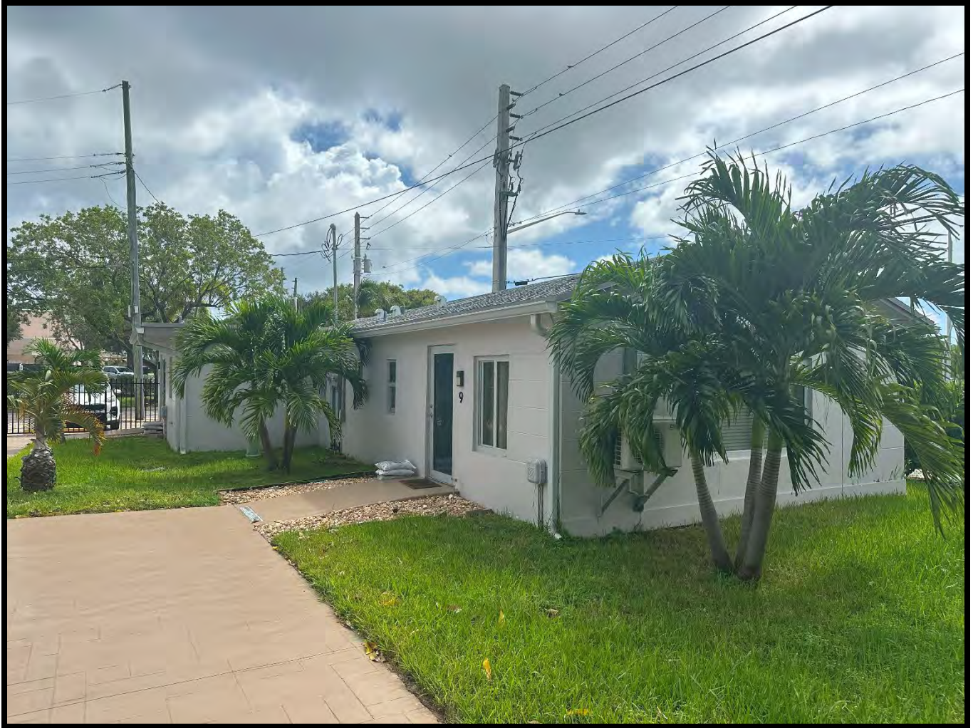
View of rear of southeast building at 414 S.E. 4 th Avenue facing easterly from courtyard
