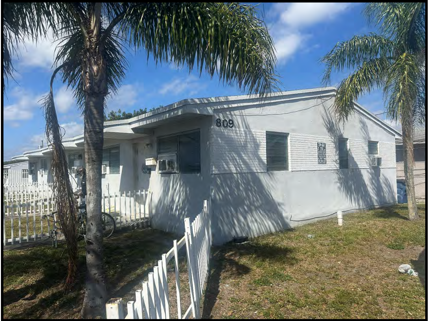
View of subject facing northwesterly from N.W. 7 th Avenue
