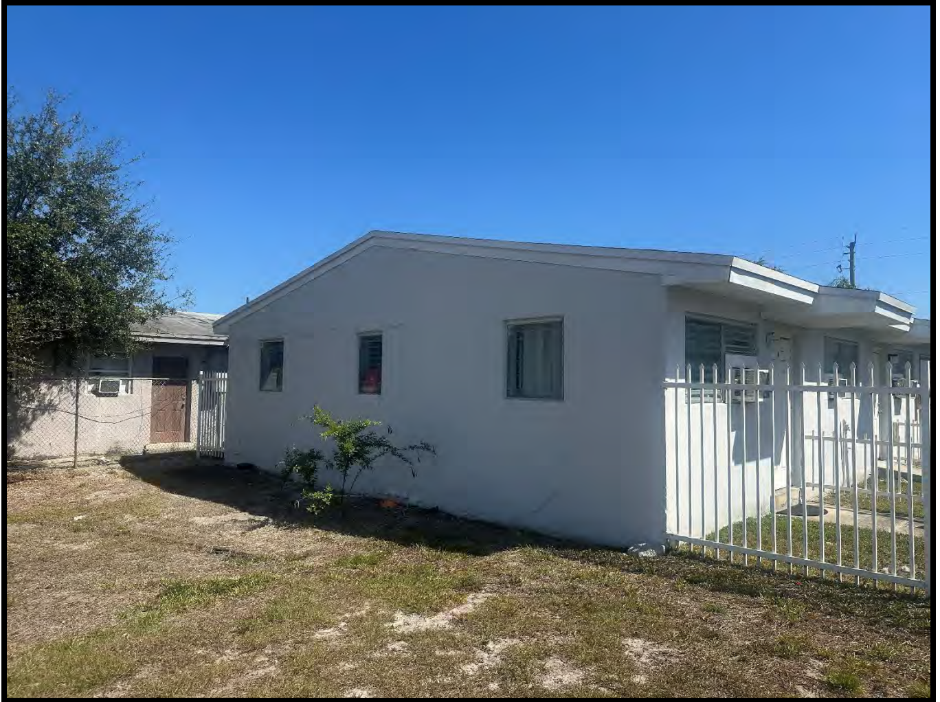
View of rear of subject property facing northeasterly
