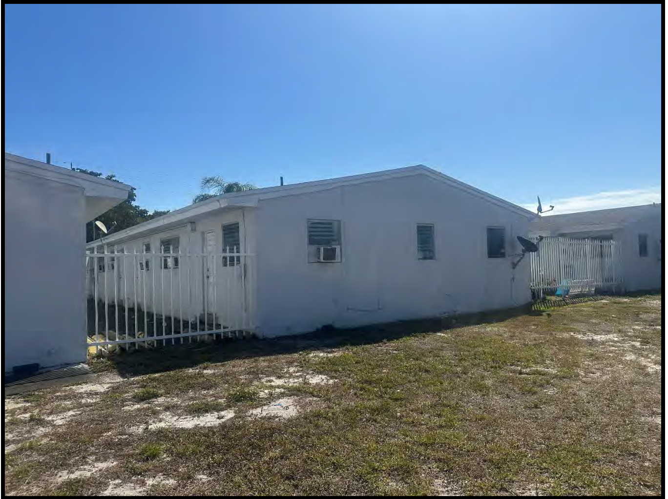
View of rear of subject property facing southeasterly
