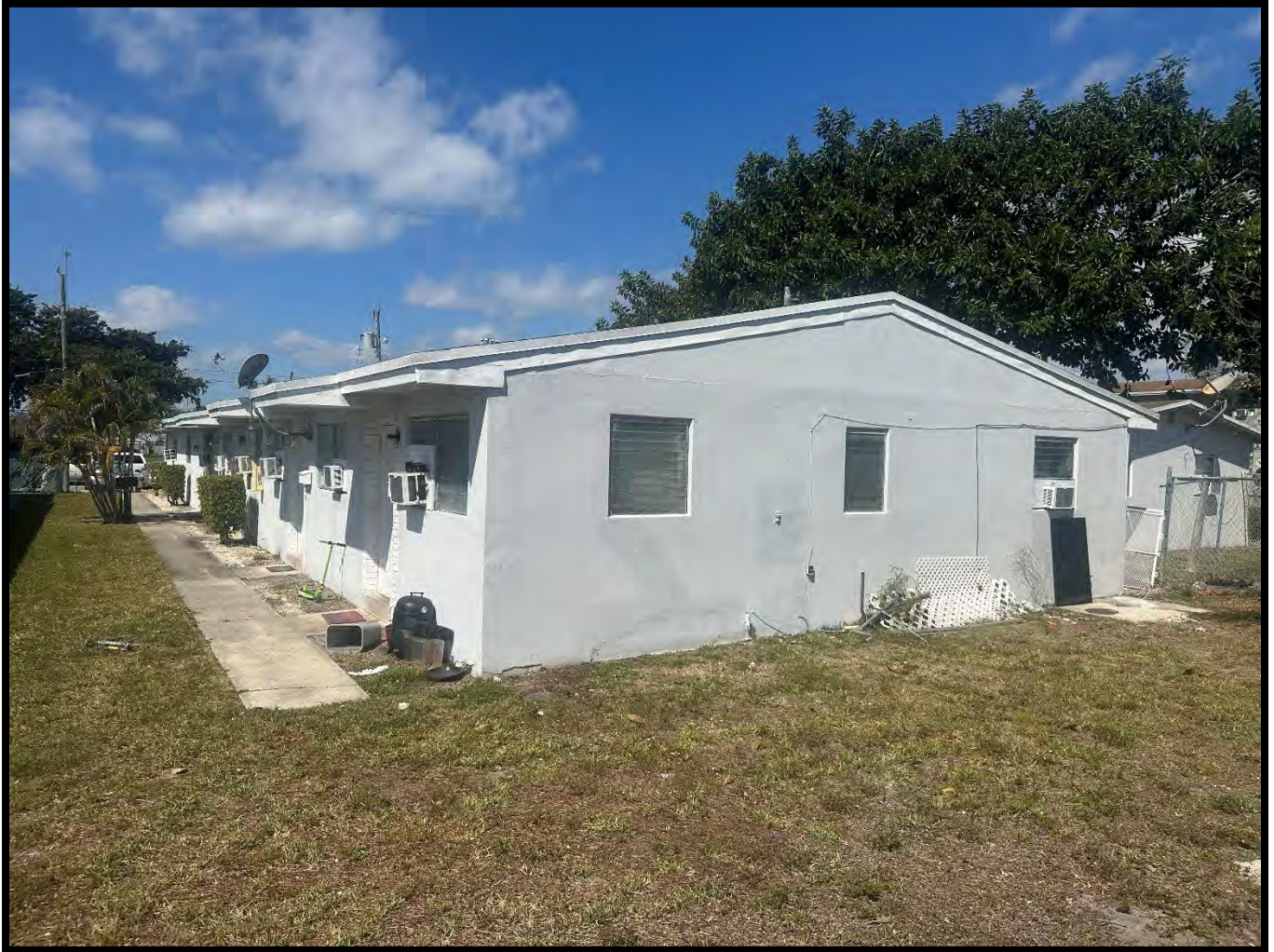
View of rear of subject property facing westerly
