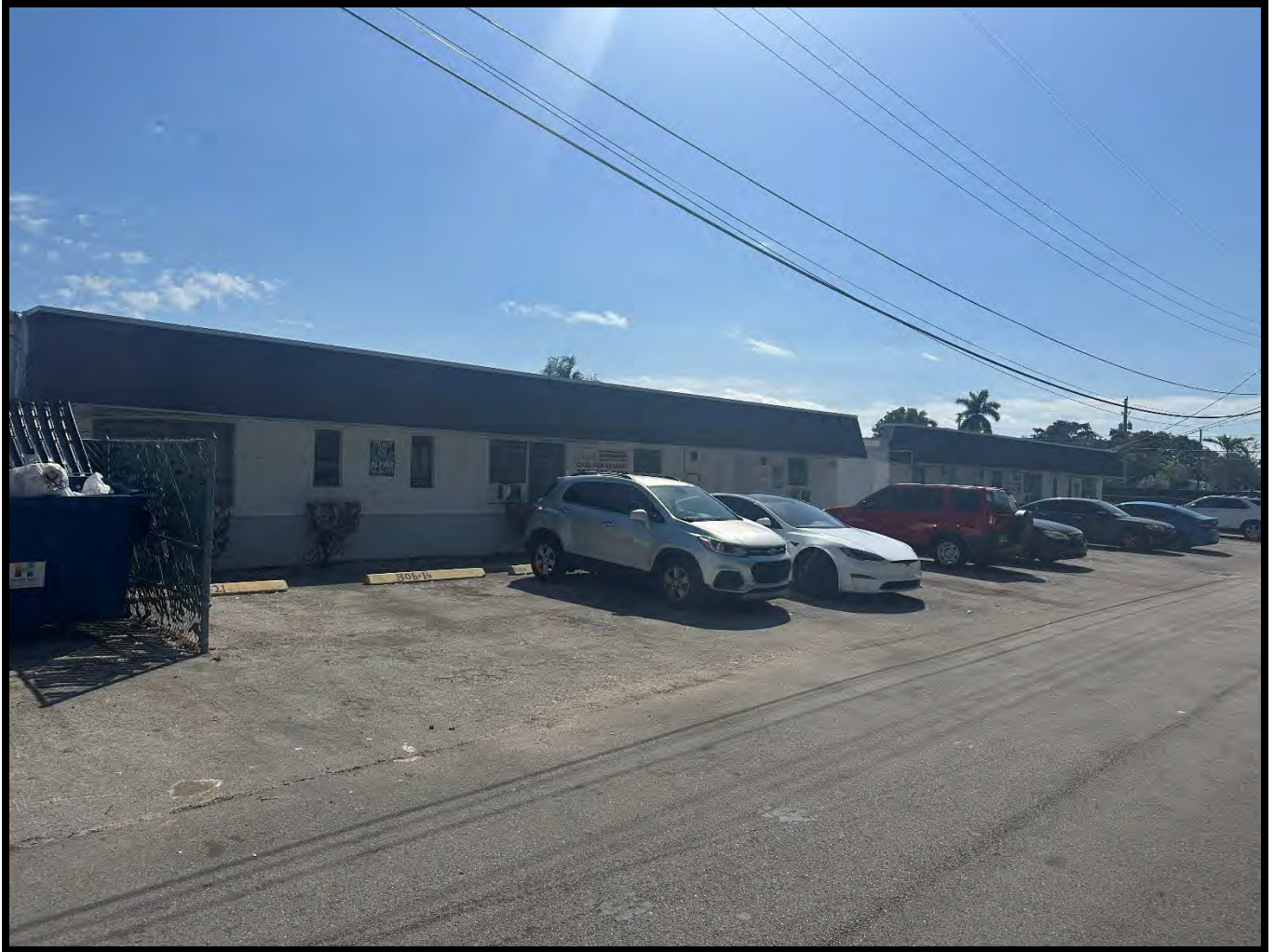
View of subject facing southeasterly from N.W. 7 th Terrace
