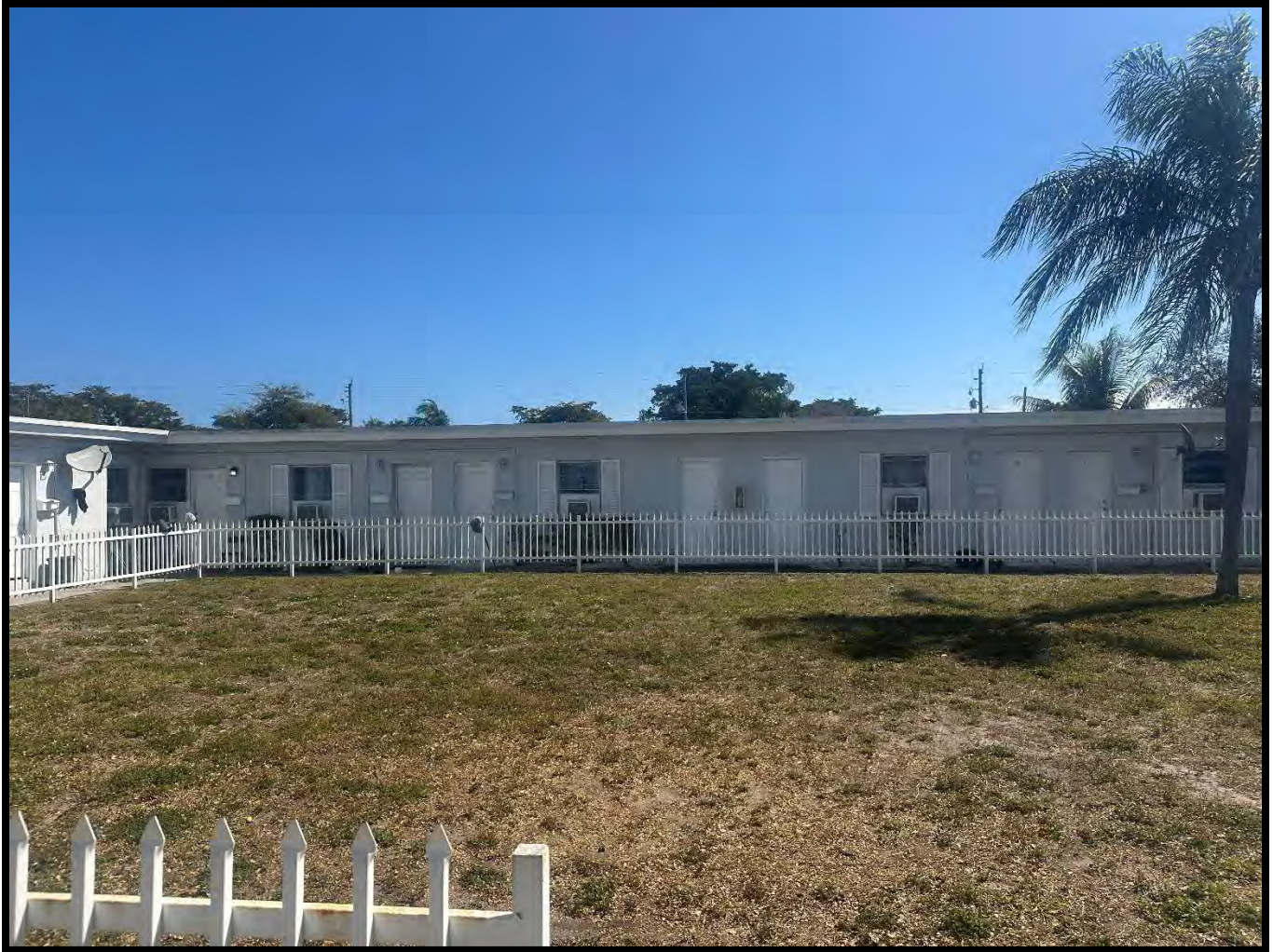
View of interior courtyard of subject property facing easterly.
