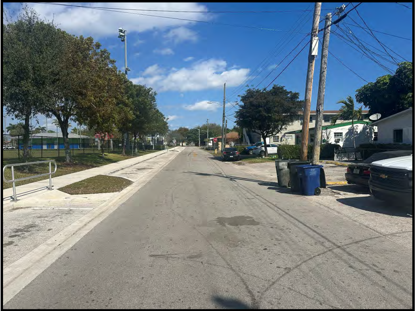
View of N.W. 7 th Terrace facing northerly with the subject on the right side. Please note that the surface-parking appears to be partially located within the existing right-of-way for N.W. 7th Terrace. The west side of N.W. 7 th Terrace has additional public parking.
