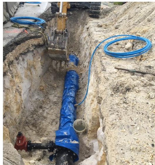
Watermain and Service Installation
