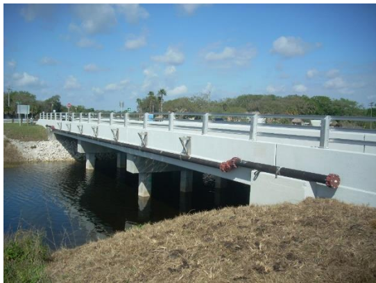
New Snake Road Bridge
