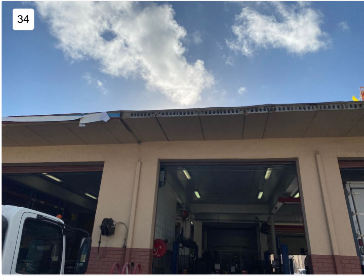
Project: #31067 Hallandale Beach - Garage Date: 7/15/2024, 8:34am Creator: Luis Becerra
