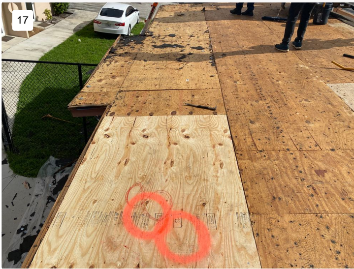
Project: #31067 Hallandale Beach - Garage Date: 6/26/2024, 9:38am Creator: Luis Becerra
