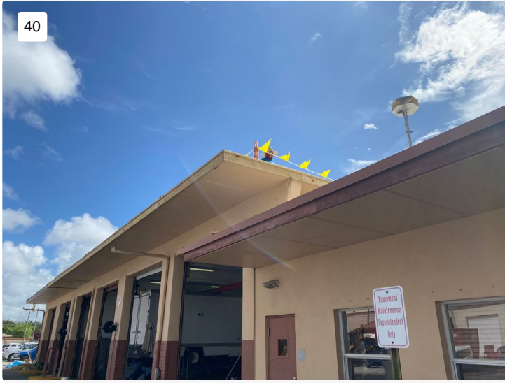
Project: #31067 Hallandale Beach - Garage Date: 7/15/2024, 10:23am Creator: Luis Becerra
