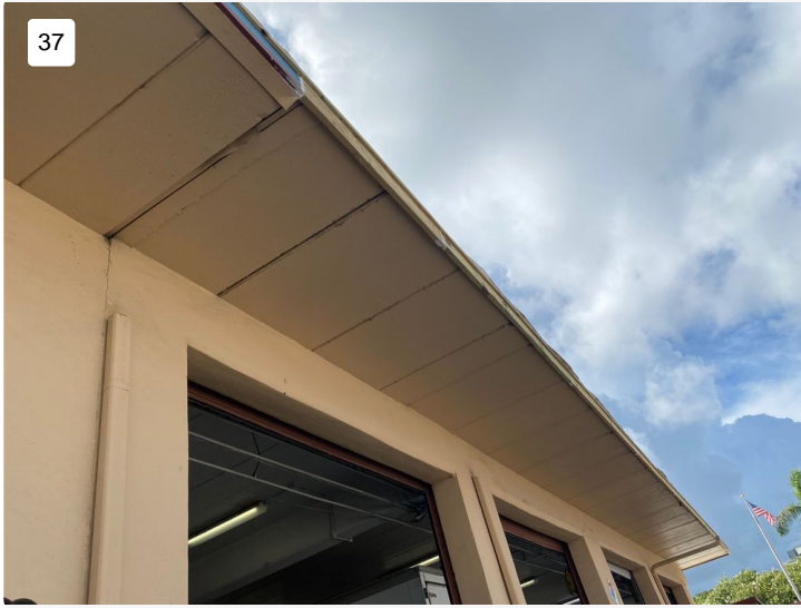
Project: #31067 Hallandale Beach - Garage Date: 7/15/2024, 10:22am Creator: Luis Becerra
