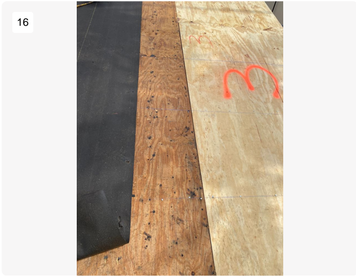
Project: #31067 Hallandale Beach - Garage Date: 6/26/2024, 9:31am Creator: Luis Becerra
