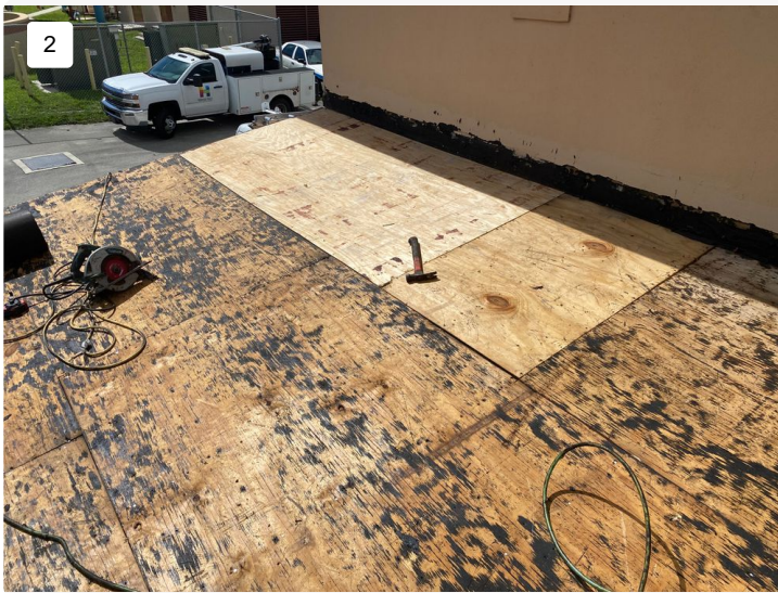
Project: #31067 Hallandale Beach - Garage Date: 6/24/2024, 10:22am Creator: Luis Becerra
