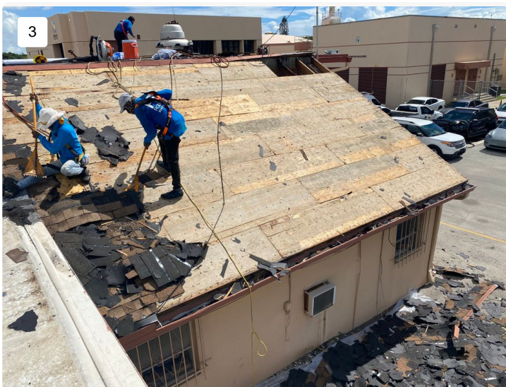
Project: #31067 Hallandale Beach - Garage Date: 6/24/2024, 10:33am Creator: Luis Becerra
