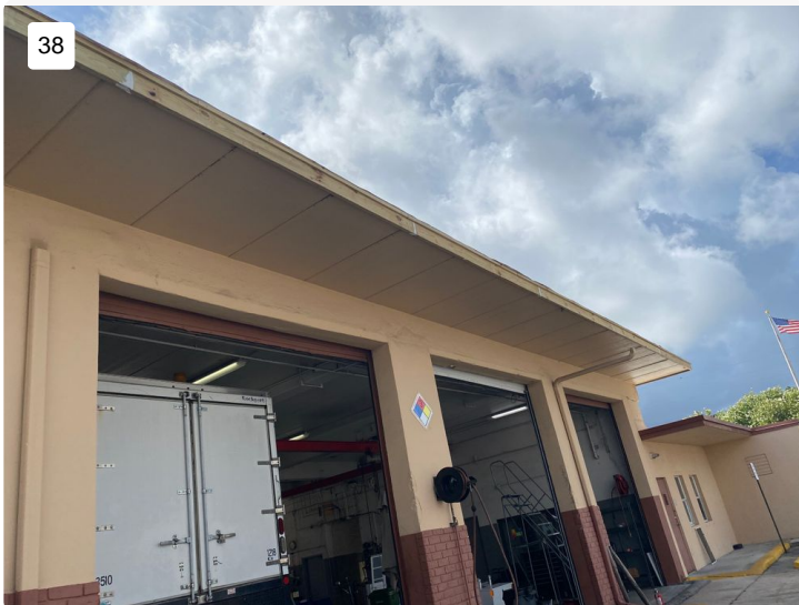
Project: #31067 Hallandale Beach - Garage Date: 7/15/2024, 10:23am Creator: Luis Becerra
