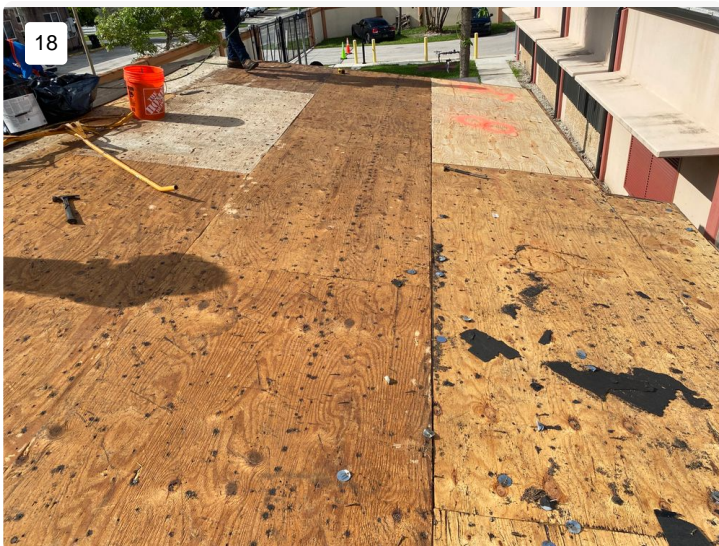
Project: #31067 Hallandale Beach - Garage Date: 6/26/2024, 9:38am Creator: Luis Becerra
