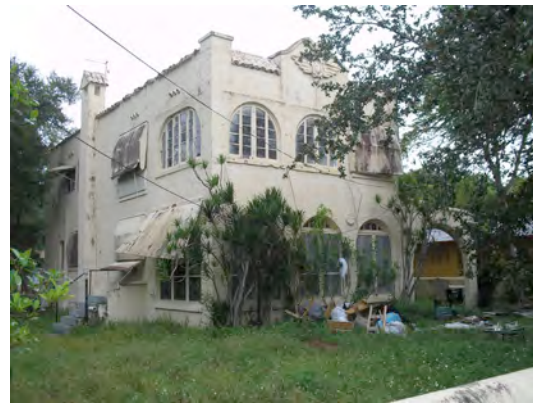
House with code problems, Southwest Quadrant
