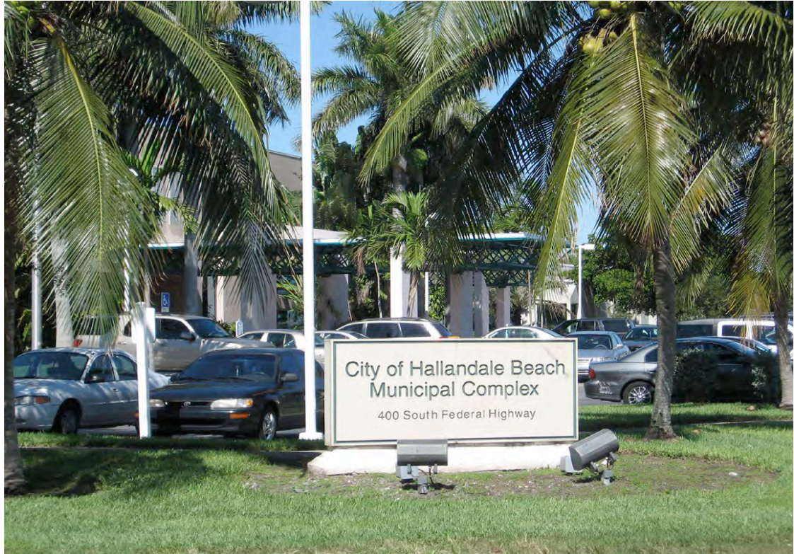
Municipal Complex, City of Hallandale Beach
