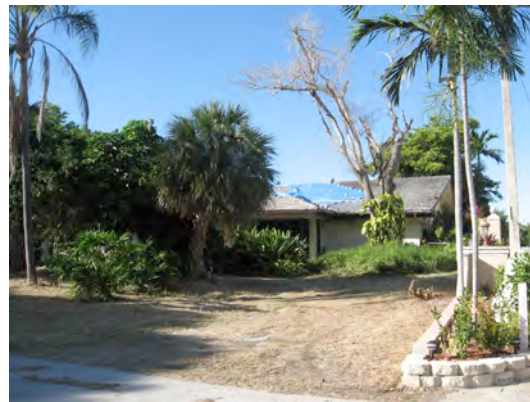
Housing with code problems, Southeast Quadrant
