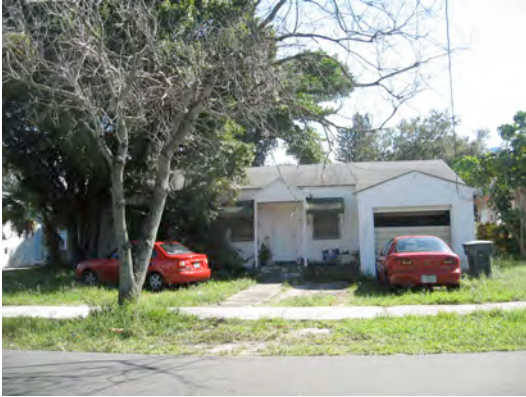
Housing with code problems, Southeast Quadrant
